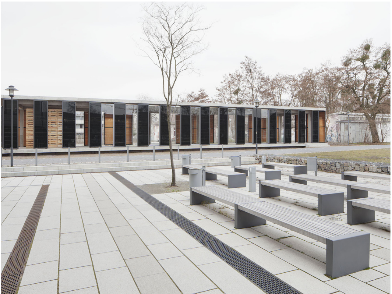
GALERIE UNTER STROM POTSDAM 2012 - Photovoltaic Pavilion FH Potsdam. The pavilion is a prototype for the integration of photovoltaic technology in space-defining architectural elements. Solar wall panels measuring four metres high and one metre wide create a façade that wraps around the 35-metre-long building. Each panel is held by a supporting steel frame. The photovoltaic elements are arranged on the outside of a continuous pane of glass. Copper switch strips can be seen from the inside, behind the glass, acting as a delicate wall cladding.
